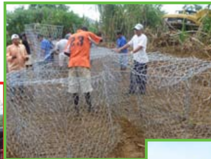
Gabions (wire mesh cages) construction
