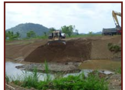
Reinforcing the river beds
