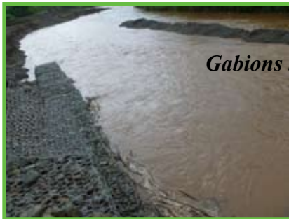
Gabions (wire mesh cages) construction
