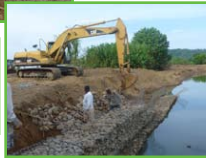
Gabions (wire mesh cages) construction
