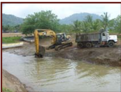
Excavating the river mud
