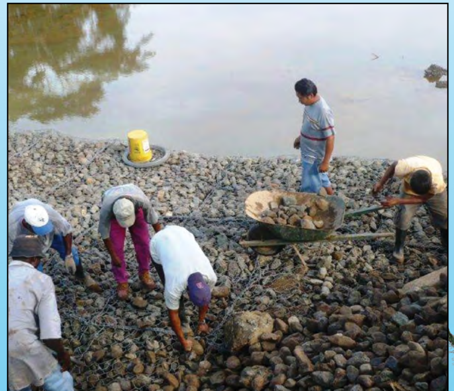
Hard at work reinforcing gabions along the rerouted Piñas River.
