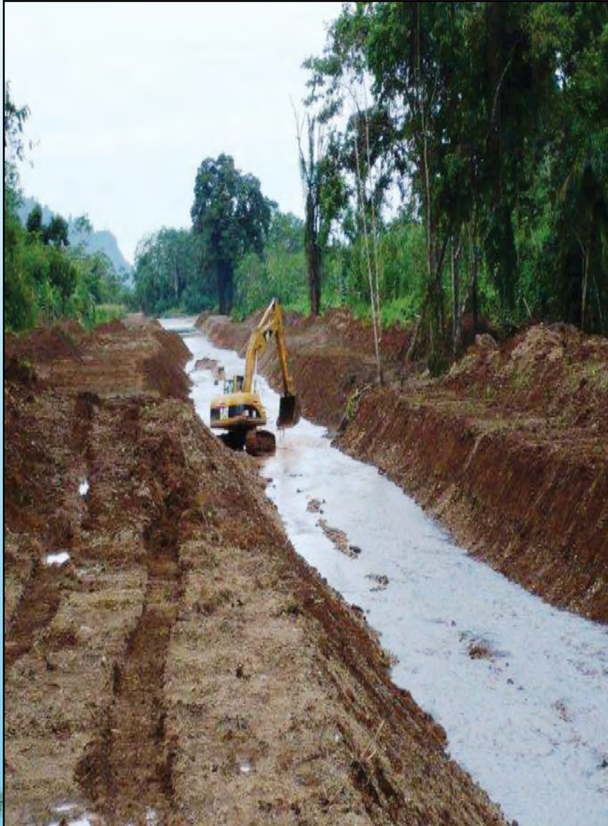
The immensity of rerouting a river is plain to see.
